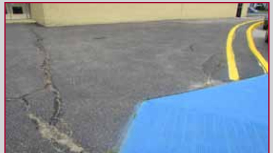
Cracked sidewalks set for repair at May Moore.
