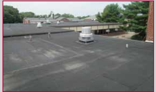
Aging roof to be replaced at John F. Kennedy Intermediate.
