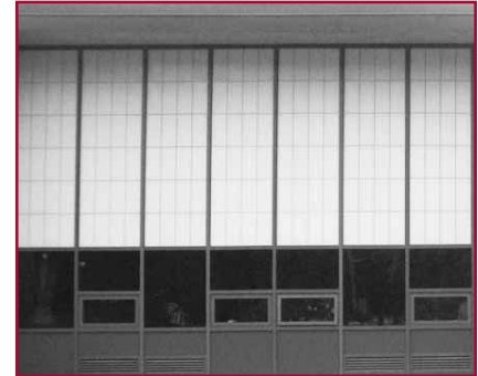
New weatherized windows line the Abraham Lincoln School.
