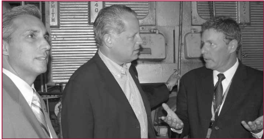
(L-R) Suffolk County Legislator Lou D'Amaro and Congressman Steve Israel visited the high school boiler room to learn from BOE President Dennis Ryan about the District's energy efficiency movement.
